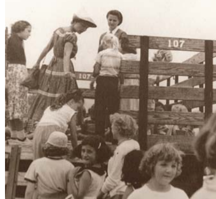
Loading the Stake bed truck (Courtesy of Bayside Community Center)
